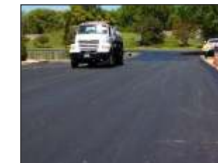
22 MILLING AND PAVING
