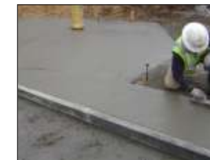
20 INSTALLATION OF GRABNET BARRIERS
