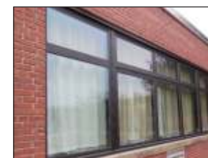
26 REPAIRS FOR BUILDINGS AT WOODLAND JOB CORPS
