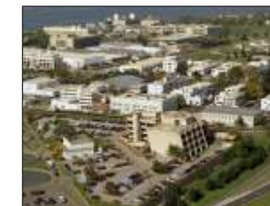
16 REPLACEMENT OF EIFS BUILDING 75
